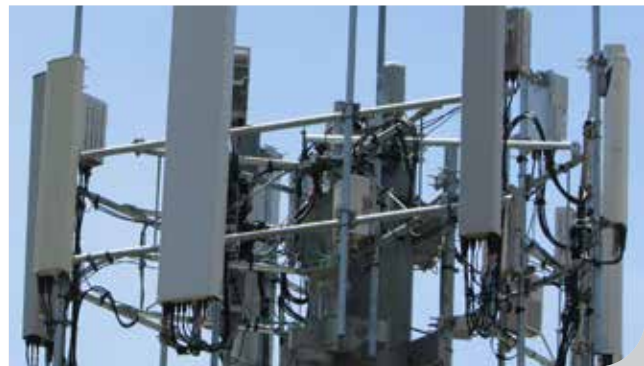
T-ARM REPLACEMENT After.
