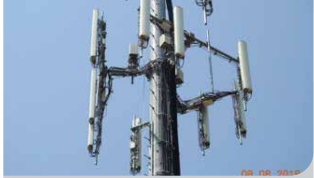
T-ARM REPLACEMENT T-arm replaced with sector frames - before.
