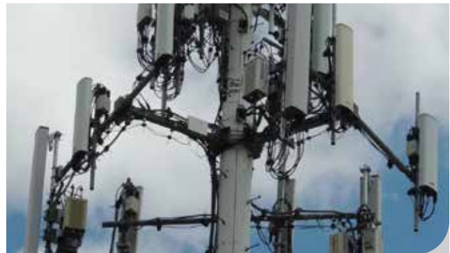
T-ARM REINFORCEMENT Before.
