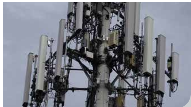
T-ARM REINFORCEMENT After.
