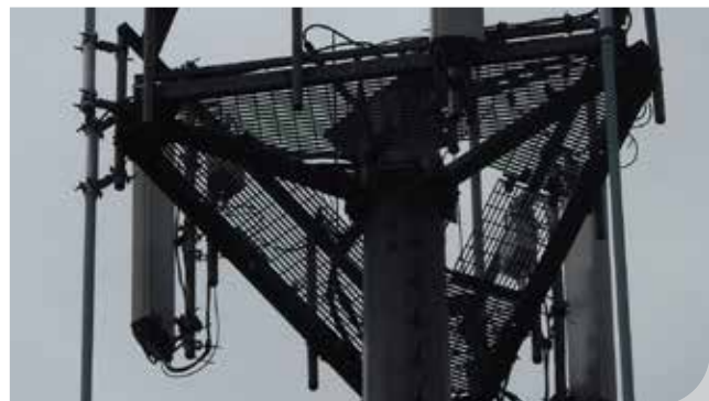
PLATFORM REPLACEMENT Before.
