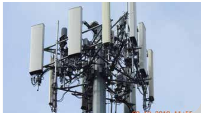
PLATFORM REPLACEMENT After.
