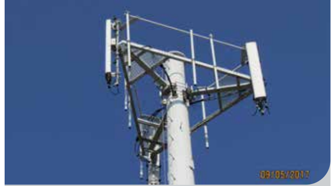
PLATFORM REPLACEMENT 3 sided platform replaced with 4 sided platform - before.
