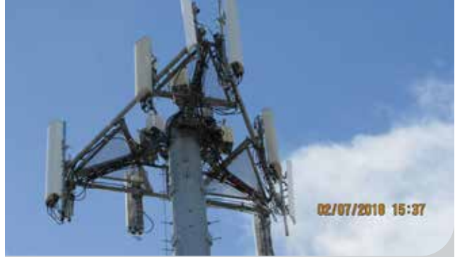
PLATFORM REINFORCEMENT Support rail addition - before.
