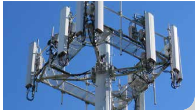
PLATFORM REPLACEMENT 3 sided platform replaced with 4 sided platform - after.
