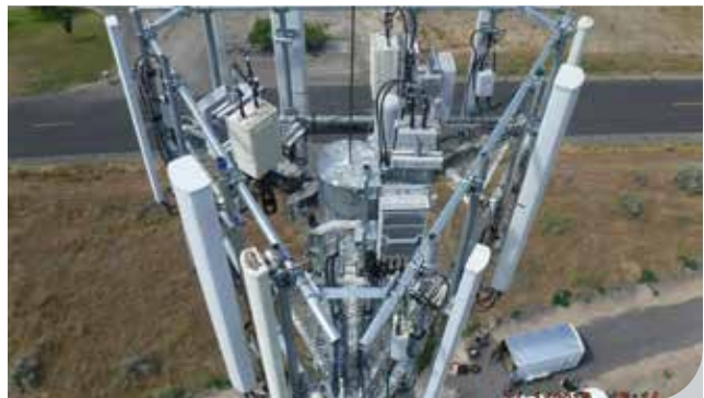
PLATFORM REINFORCEMENT Support rail addition - after.
