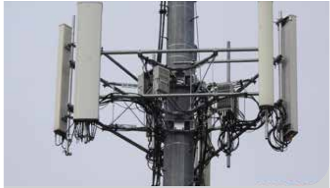
T-ARM REPLACEMENT T-arm replaced with sector frames - after.
