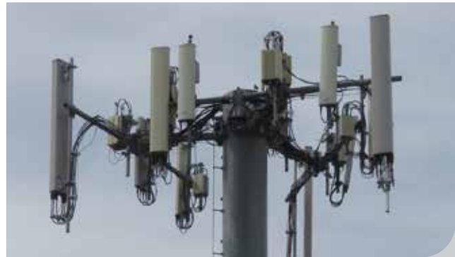
T-ARM REPLACEMENT Before.
